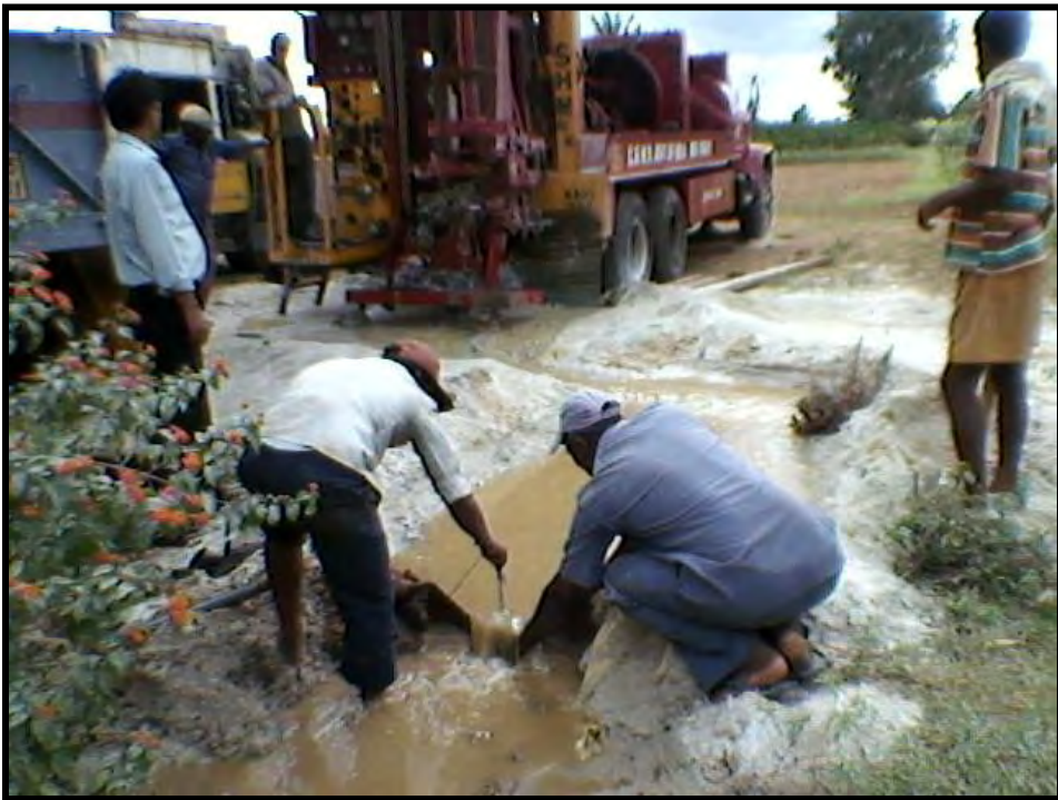
Fig 4.8 Discharge measurement of high yielding well at KOLAR DISTRICT Karnataka
